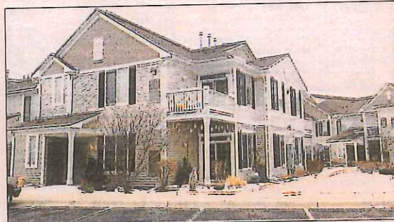
Prairie Brook Apartments at Farmington Lakes in west suburban Oswego has 304 units in 19 two-story buildings. Residences are set on a 17.5 acre site.
